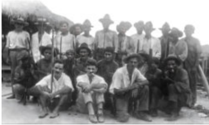
The 10 men standing in white shirts are probably workers from The Colon Development Company (TCDC) and the 11 men in dark shirts, both standing and crouching, are Standard Oil Company of Venezuela (SOV) "Militians" Seated from left to right: E. Moriarty, A. Oeuvray, E. Edwards, and probably P. Torres.
